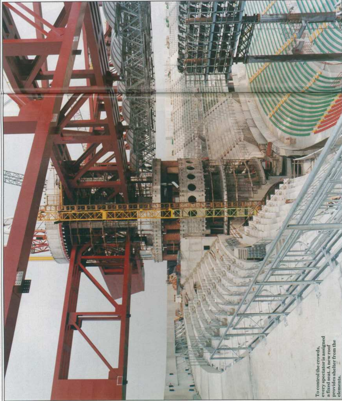
A new roof of polycarbonate-barrel-vaulted units is supported on a colossal steel structural frame.
