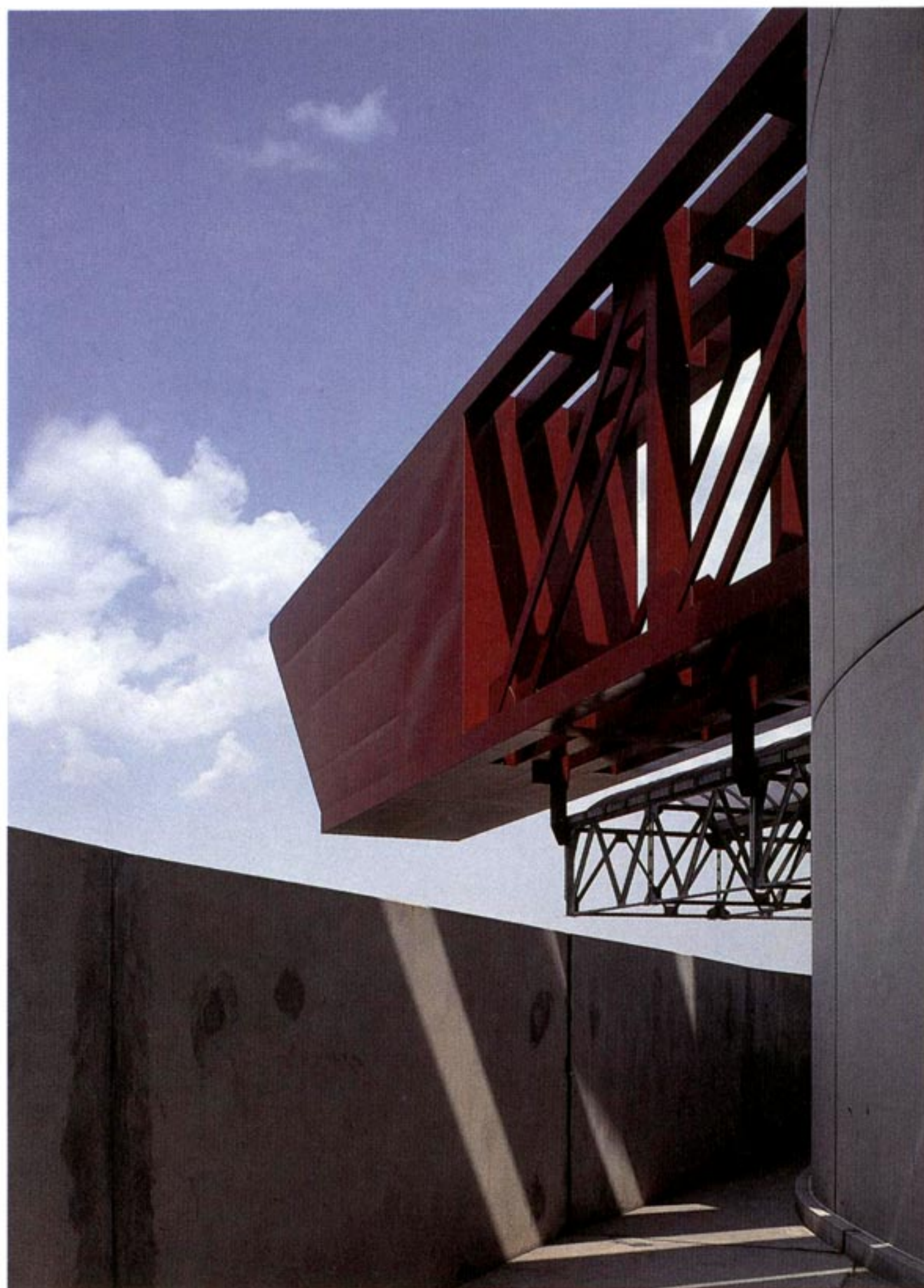
(above:left to right) Detail of the top structure: Detail of the high corner tower and the enormous pylon beams. Detail of the trussed beams bearing the roof. Detail of the trussed beam and the roof structure—a spatial grid system containing small translucent polycarbonate vaults. Upward view with trussed beam, roof and new tiers.
